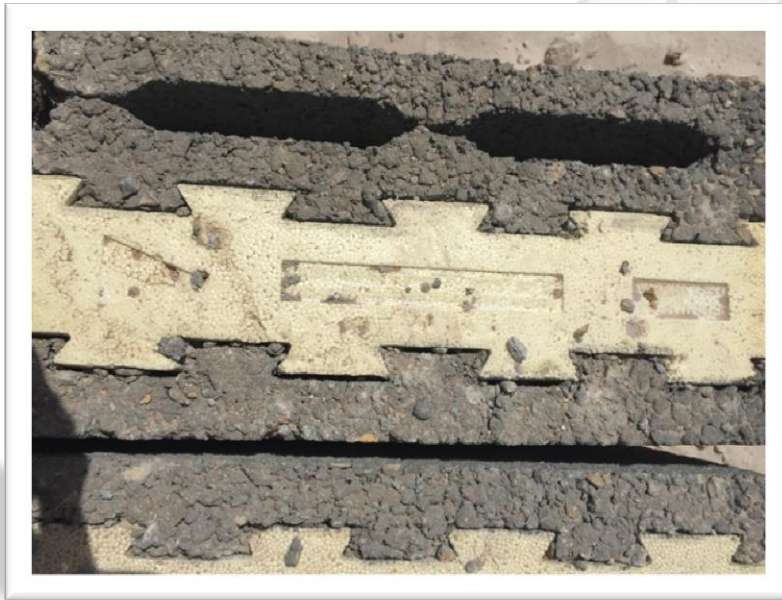
1- With Polystyrene Insulation
